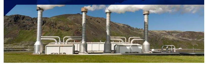
In high pressure and temperature geothermal wells geothermal water is extracted and flashed in a separation vessel. The flashed steam is used for power generation in a steam turbine. The remaining geothermal water still has high temperatures often in the range of 160°C. This water has still a high potential for power generation in a ORC where a working fluid is evaporated which is later expanded in a turbine. While evaporating the working fluid the geothermal water cools down.
